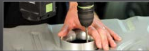
Use installation ring to locate mount holes
