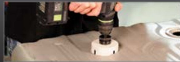
Drill 3.25in hole in the deepest spot of the tank
